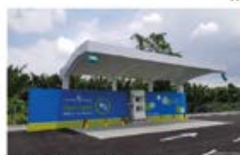
Hydrogen Refueling Station
